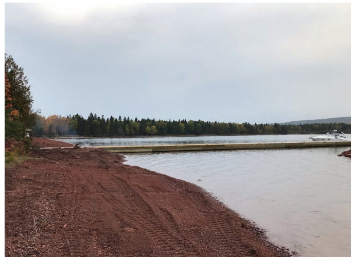
Rebuilt Siskiwit Bay Dock - Steve Hanke
